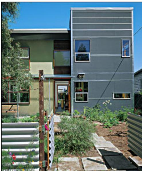
The exterior is finished with Hardipanel, placed vertically on one volume and horizontally on the other. The house numbers are neon that glow red-orange at night.
