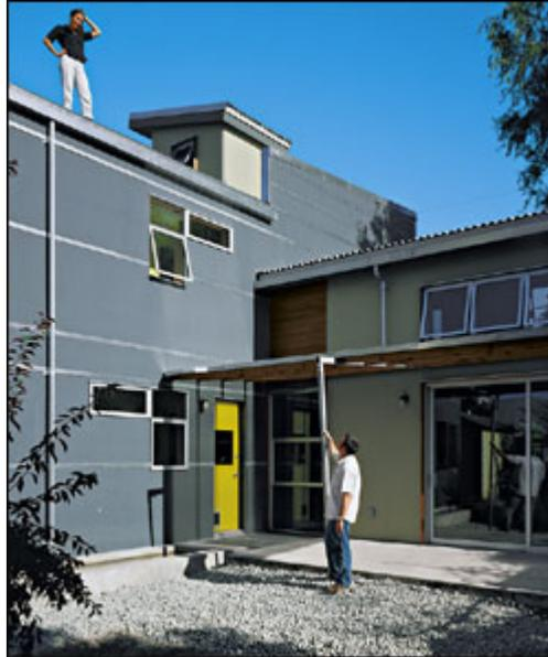
The roof drainpipe empties into a rectangular reflecting pool. It's part of the water-catchment system, which stores runoff in a 1,200-gallon underground cistern. The system is an example of sustainable building practices that the couple incorporated into their home, and that are increasingly inspiring architects.
