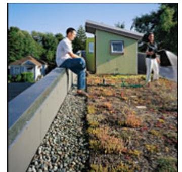
The living roof has about 4 inches of lightweight soil. Trial and error have led the couple to concentrate on sedums and creeping thyme. The living roof reduces heat reflection, and slows and filters storm-water runoff.
